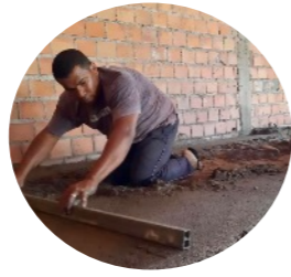
Gaditas Training Center construction
