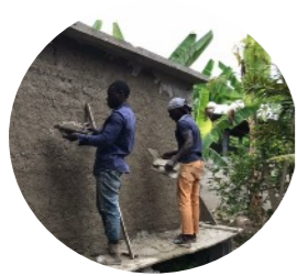
Haiti Resource Center construction
