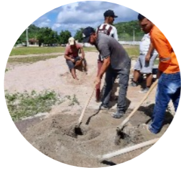
Sertão Training Center construction
